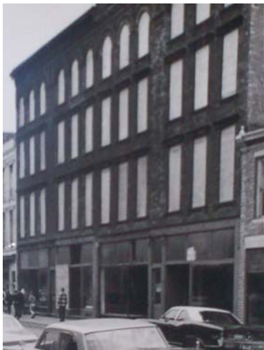
The Coatsworth building with windows boarded up to keep the 'coons and pigeons out. (plhc)
